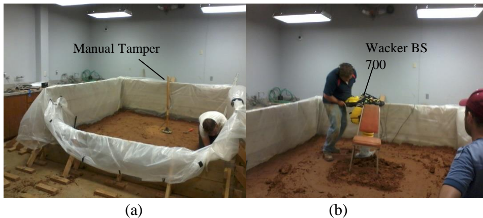
Figure 3.3. (a) Manual tamper on center of pad, (b) Wacker near the center of pad.
